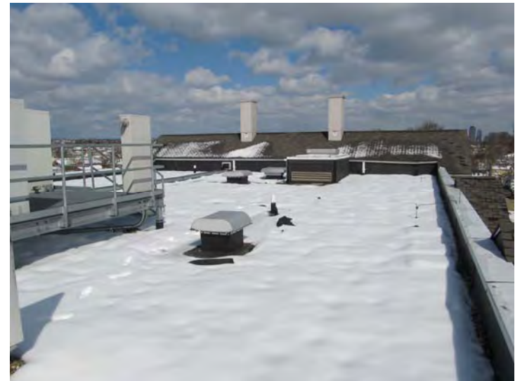
Flat roof section features an original adhered membrane covering
