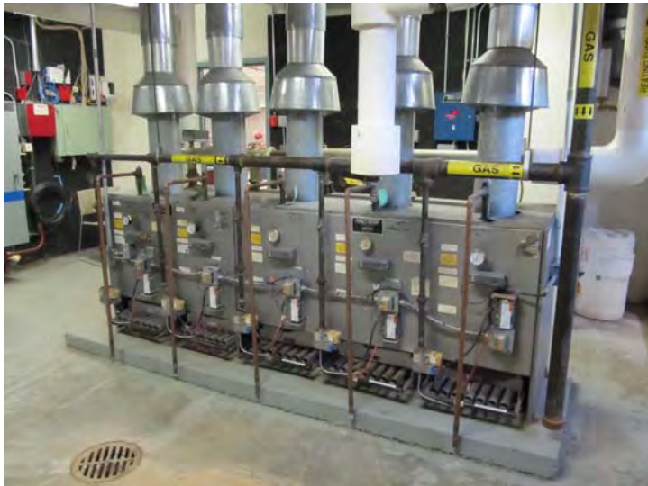
Hydronic heat for the facility is produced by an original, Hydrotherm, natural gas-fired modular boiler plant
