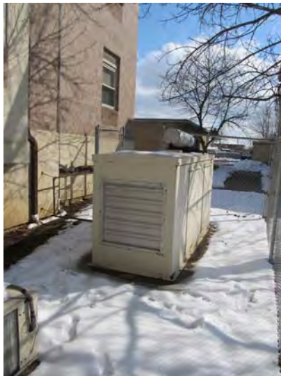
Original, natural gas-fired, generator provides emergency power for select components/systems
