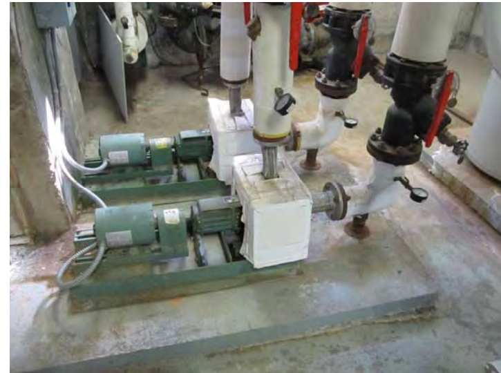
Base-mounted circulation pumps for distribution of hydronic heat
