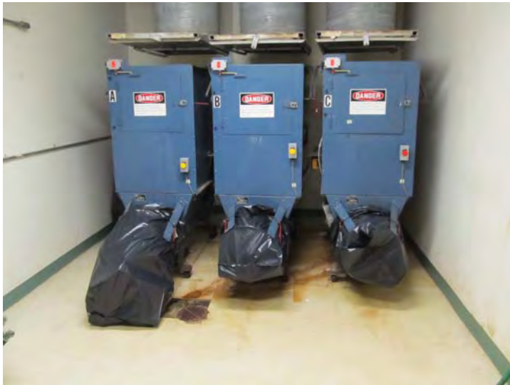
Original chute-fed sausage bag waste compactor units – No problems observed or reported
