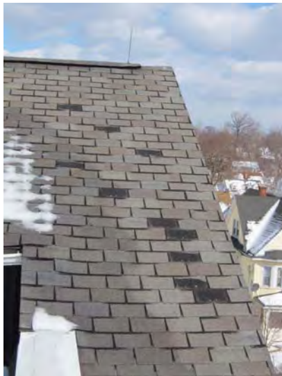
Missing/broken original shingles noted at various locations on pitched sections of roof surface
