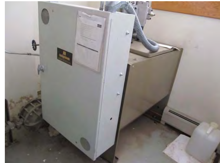
Original hydro-mechanical and controller/dispatcher equipment for elevator – Full service contract in place and no problems observed or reported
