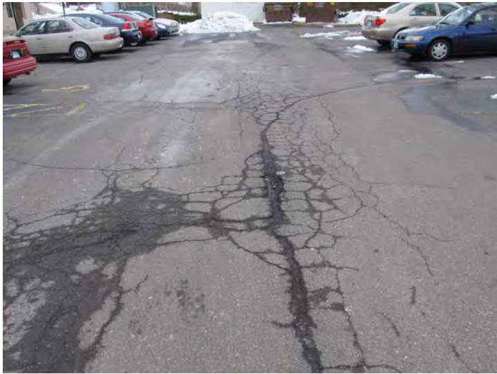
Asphalt paving in parking area starting to exhibit age-related cracks and deterioration
