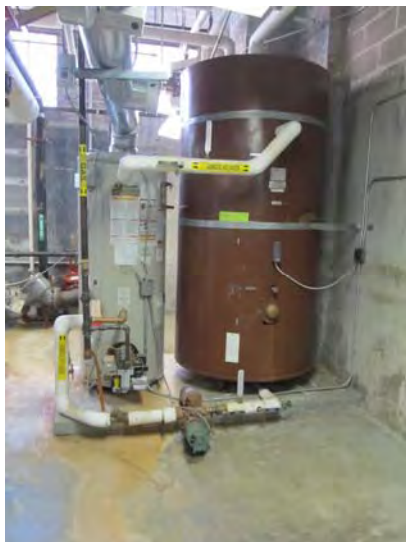
Freestanding natural gas-fired domestic hot water tank (on left) and adjacent 500-gallon storage tank
