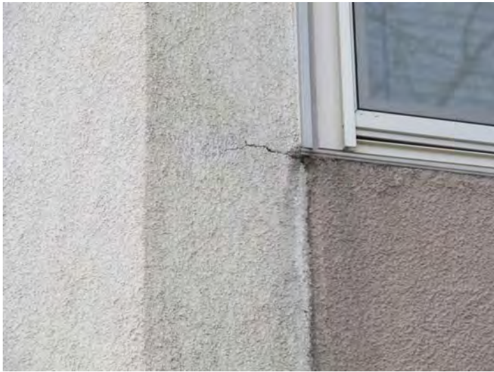
Cracks noted in EIFS at some locations
