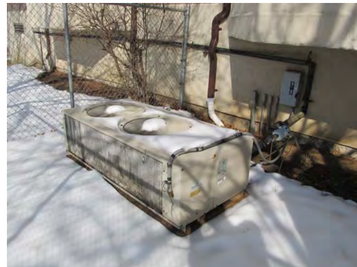
Original exterior condenser unit provides cooling capacity for select interior common areas
